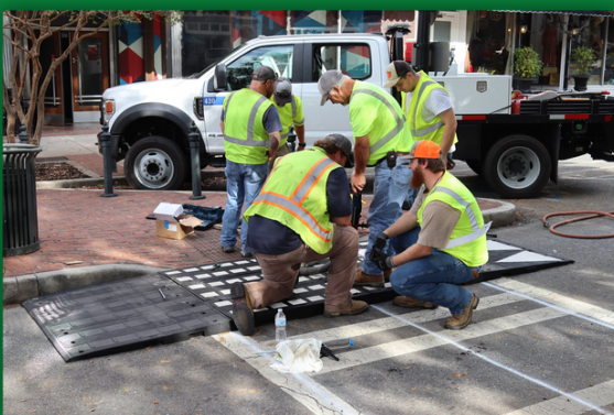
Speed Tables installed at mid-block crosswalks up and down Broad Street
